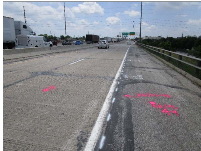
Figure 2-4: Deteriorated Pavement Conditions
