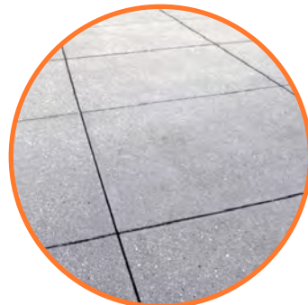
SAW CUT JOINTS
